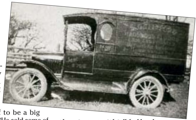
Above: Contractor Sid Galliford bought his first work truck in 1923 — a Ford Model T. Right: No electricity was required for this early-1900's version of a sanding machine.
